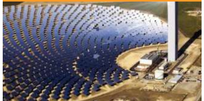
POWER TOWER + HELIOSTATS
