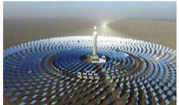
Concentrated Solar Power
