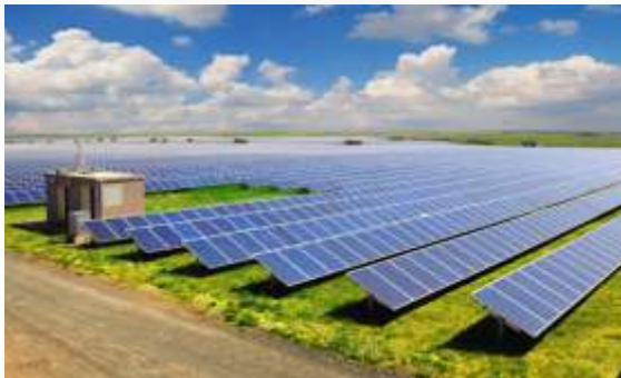
Photovoltaic Panel Solar Farm
