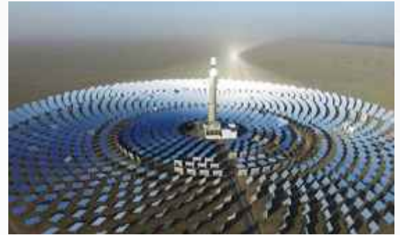
Concentrated Solar Power
