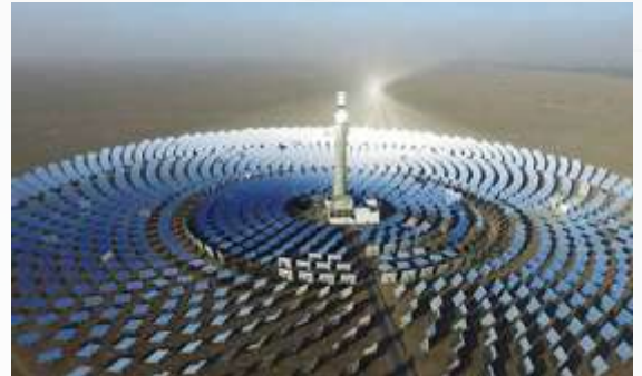
Concentrated Solar Power
